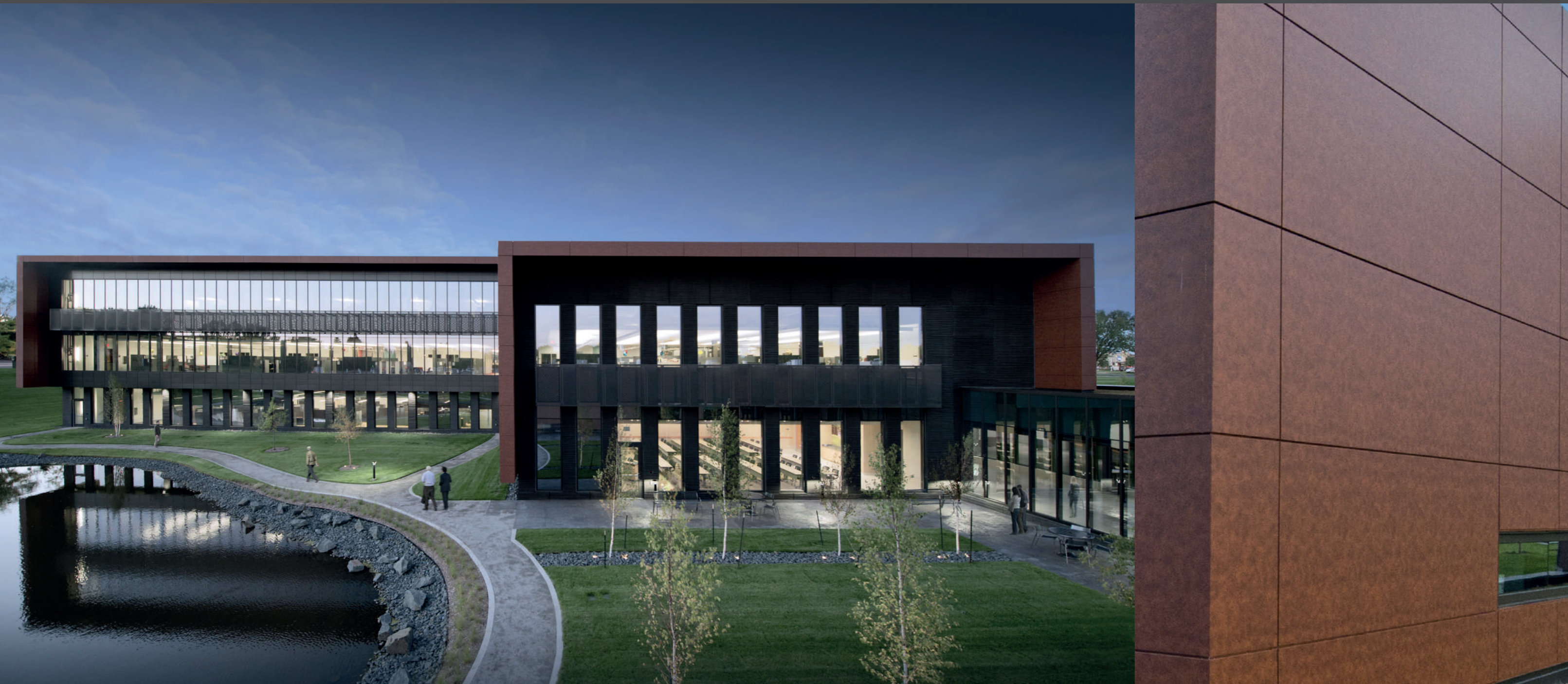
Toro Headquarters | Minnesota | U.S.A
