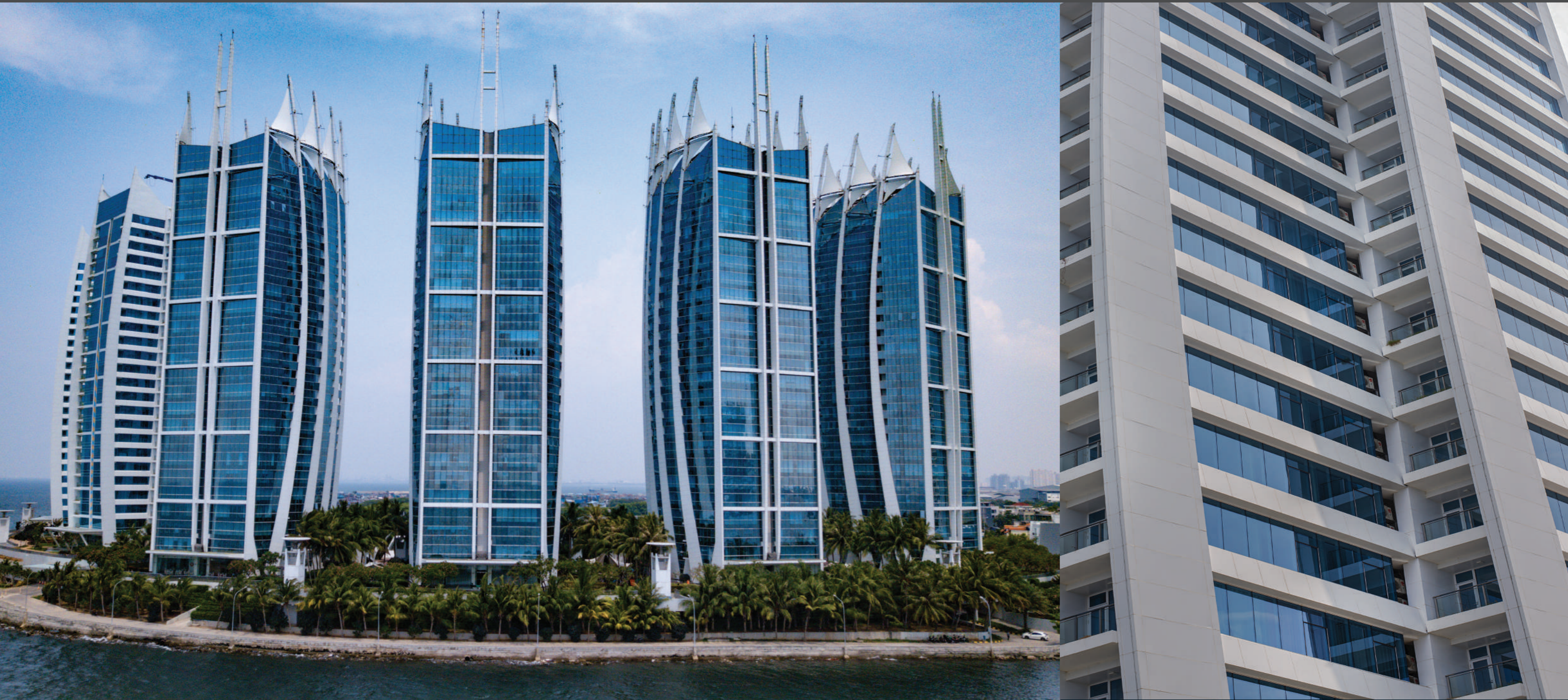
Regatta Condominium | Jakarta | Indonesia
